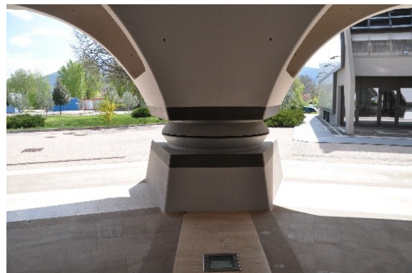
The centre's buildings are all earthquake-safe; entrance to the centre - one of the pillars with flexibility
